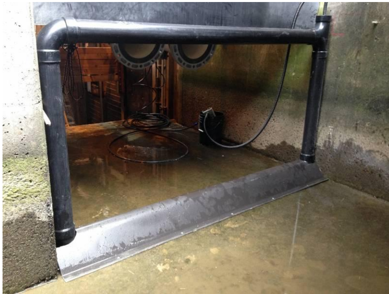
Figure 3. Antenna positioned near the entrance to the exit channel to confirm results from earlier noise listening effort. Fiberglass (FRP) ramps would be used to reduce flow disruption. This location did not result in noise on the BO3 system, but did raise concerns about possible fish strikes and flow disruption.
