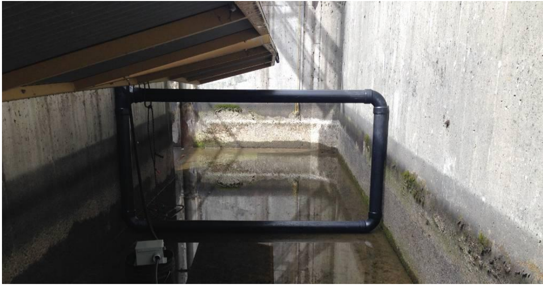
Figure 1. Antenna placed at proposed alternative location. Antenna at this location resulted in elevated noise levels on the existing BO3 system.
